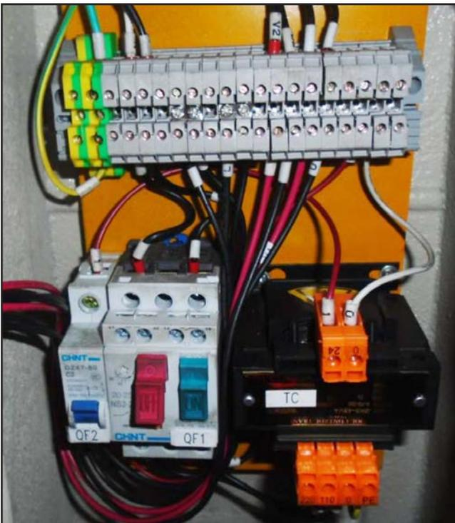
Figure 83. G0802 electrical panel wiring.
