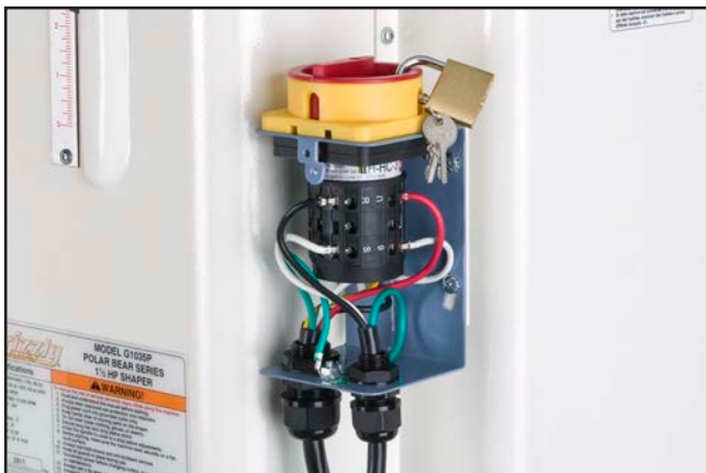
Figure 79. FWD/REV switch wiring.
