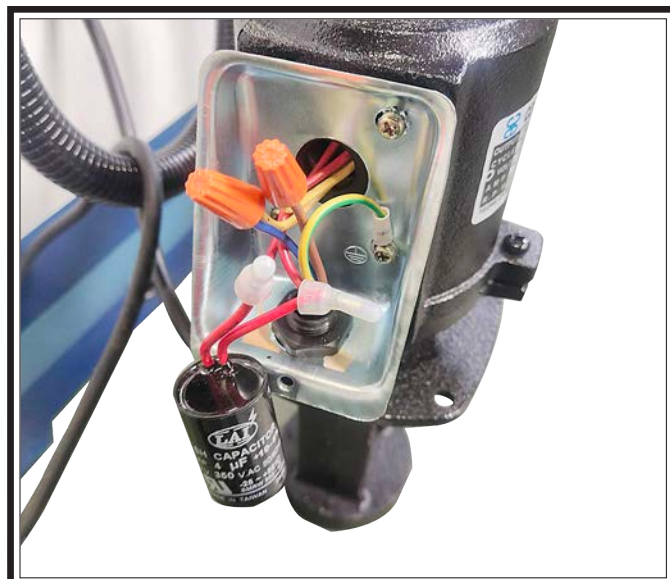
Figure 70. Coolant pump motor wiring.
